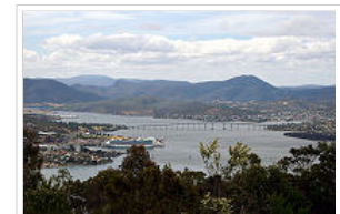
Tasman Bridge from Mount Nelson
