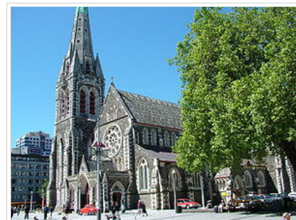
The Anglican cathedral was completed in 1904 and has since been the focal point of the city
